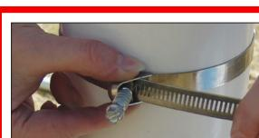
**DO NOT use a power tool to tighten the stainless steel bands! Over tightening will cause damage.**
