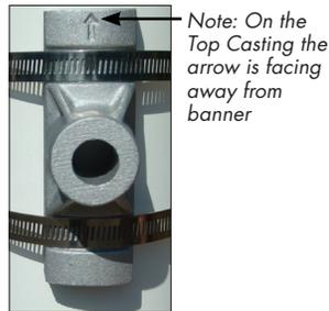
Secure the top Casting (1) to the Pole with two Stainless Steel bands (3). If attaching to a square or other shaped pole, it is recommended to use an additional set of bands, available separately. Tighten the bands until they hold the bracket securely and lock it into place with a screw or nut driver. Be sure the Band head is on the side of the pole and not on the casting. Clip off any excess band length.
